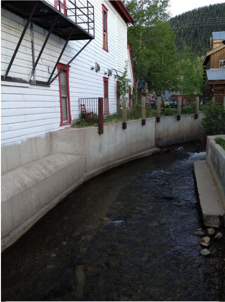
A flood wall along Coal Creek mitigates flooding in Crested Butte. Photo J. Brislawn 6/2012
